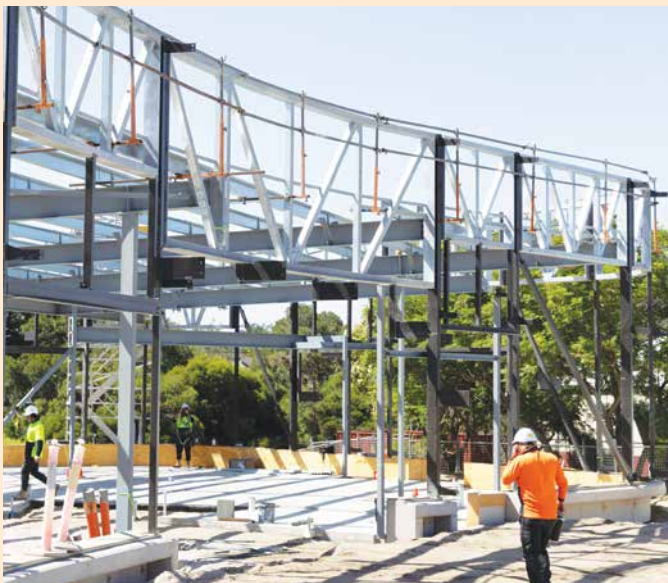
Construction is underway at Dordaak Kepup.
