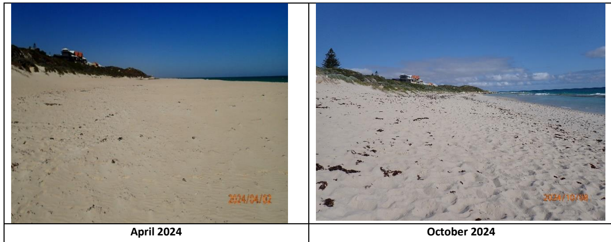
Figure 4-8 Major erosion over winter 2024 at Yanchep B08 Down-Coast.
