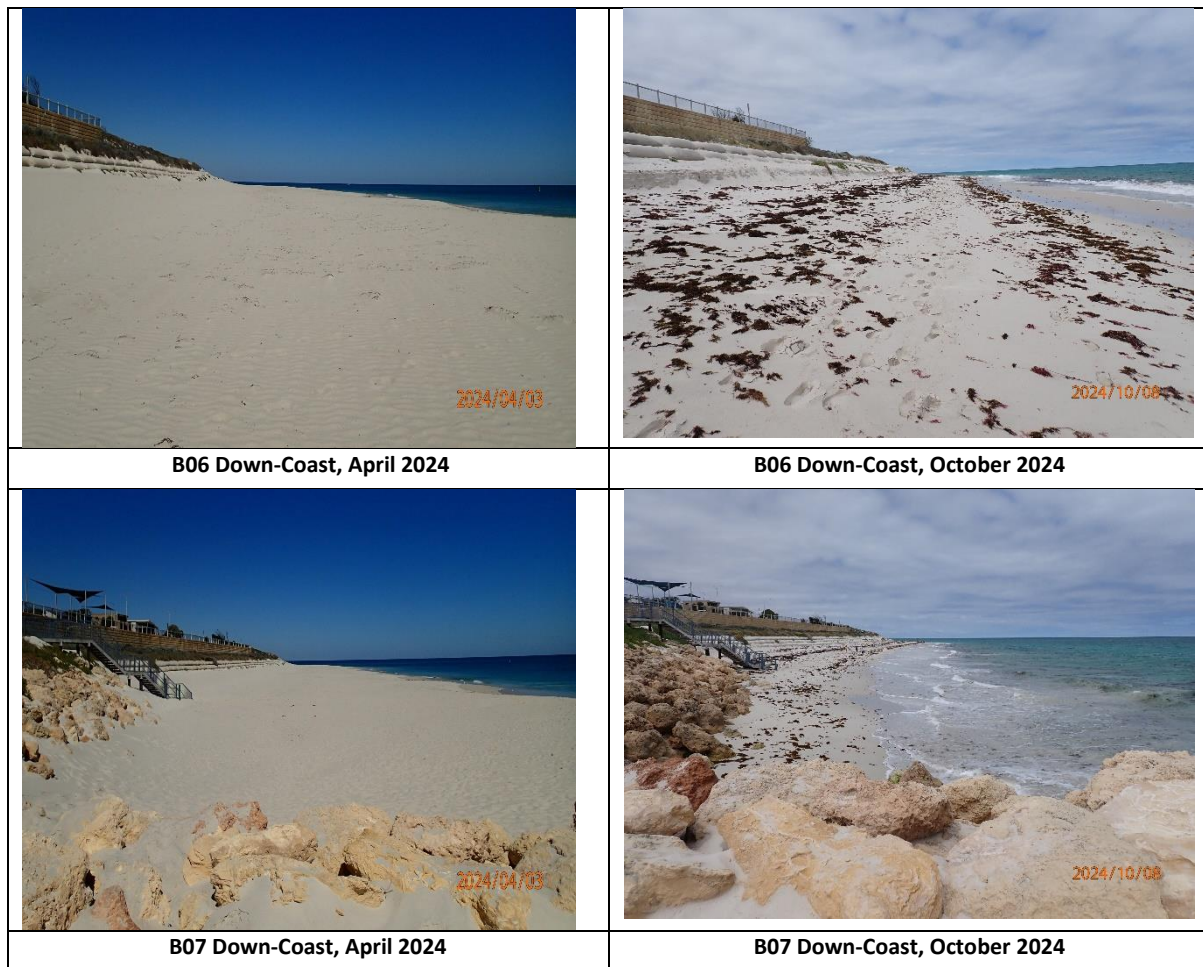
Figure 4-10 Major erosion over winter 2024 at Quinns Rocks Rock B06 and B07 Down-Coast.
