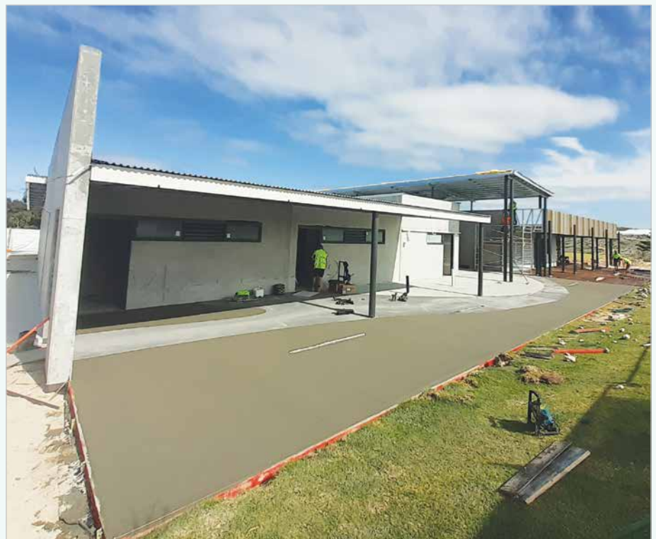
Heath Park Pavilion construction progress, October 2024.
