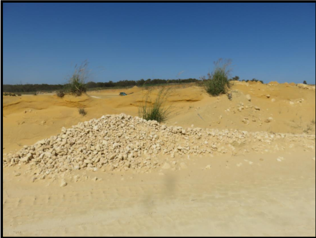
Photo 6: Sparse Grassy Weeds in Excavation Footprint
