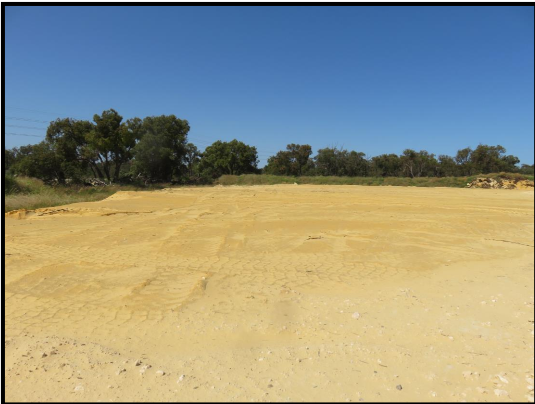
Photo 4: Finished Levels at Proposed Site Office Location
