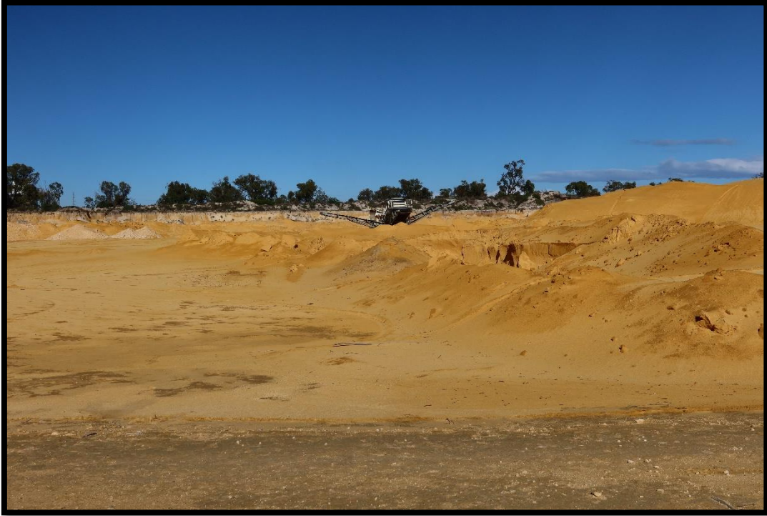
Photo 1: Excavation east of Mather Drive
