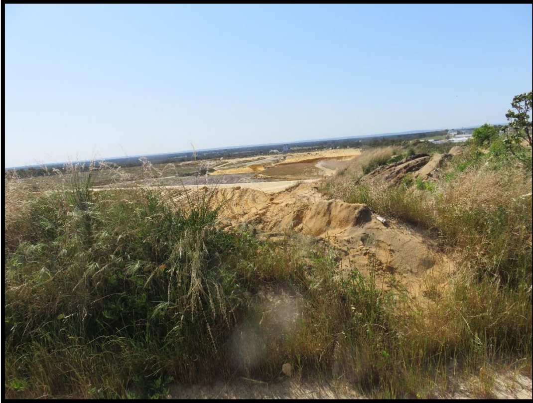
Photo 1: Excavation east of Mather Drive
