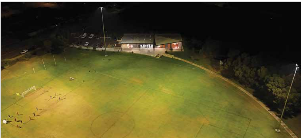
New floodlighting in action at Dalvik Park, Merriwa.
