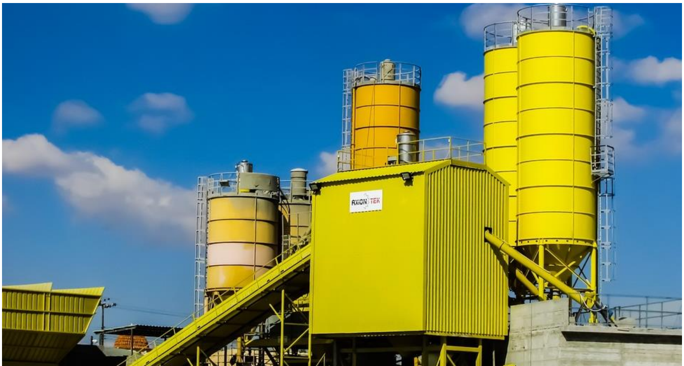
Figure 2-1 A typical concrete production facility, which comprises several energy-intensive processes.
